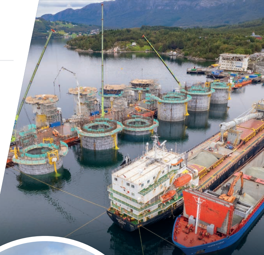
construction of the project's 11 floating concrete hulls underway at Dommersnes
